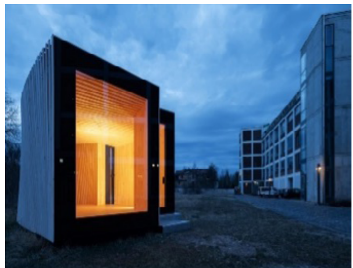
Timber prototype house: A solid wood box with 15m 2 of interior space to test the practicality of this construction method. (Credits: IBA Thüringen / Thomas Müller)
